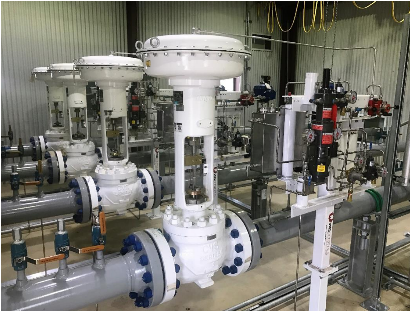
Louisville Gas & Electric (LG&E) CVET Globe Control Valves with VPC Valve Pilot Controllers w/ VMO
